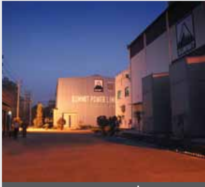
ASHULIA POWER PLANT | 44.75 MW
