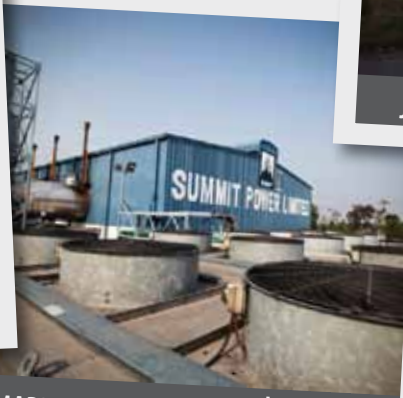
MADHABDI POWER PLANT | 35.30 MW
