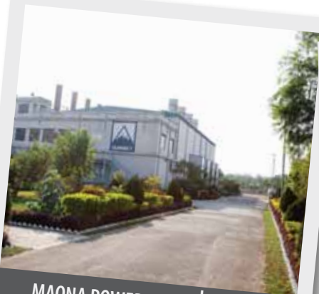
MAONA POWER PLANT | 33 MW
